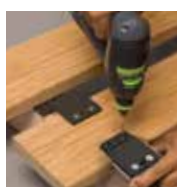
Pre-drill with the template
