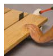
Mount the final board
