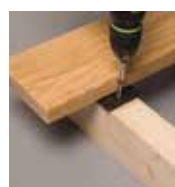
Fasten to the joists with screws
