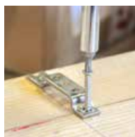
2) Mount KOMBI bracket with screws
