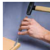
4) Knock in with the insert tool
