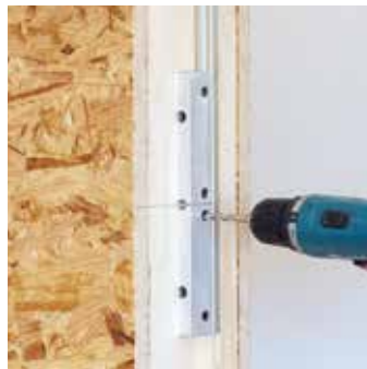
1) Predrilling with drilling-jig
