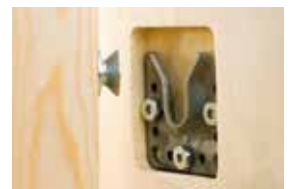
Installation example: Mounted on the wall element.
