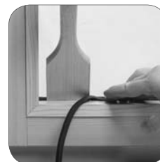
5. Press in wedge-shaped sealing
