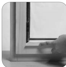
4. Snap in glazing bead
