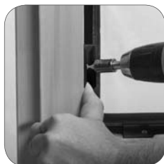
3. Fix FIXclip GLE20 Plus and set pressure with 45° slanted screws
