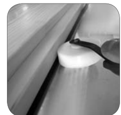
6. Clean finish with usual sealing roller
