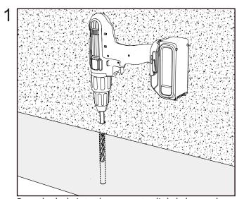
Bore the hole into the concrete slightly larger than the external steel thread, taking note of the depth required.
