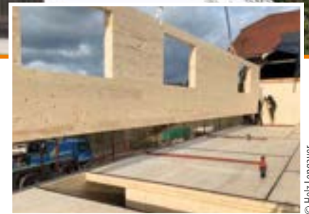
Installation example: CLT walls installation.
