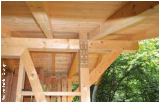
With T-JOINT D35 W30 fastened hardwood tension ties for BSH tension joints.
