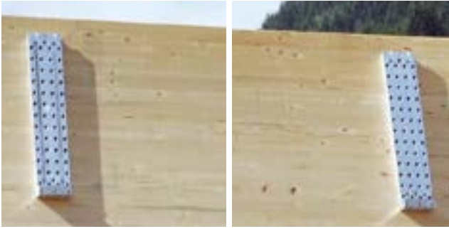
With only 2 cm of hooking way, an installation in recesses of concrete walls can be done.
