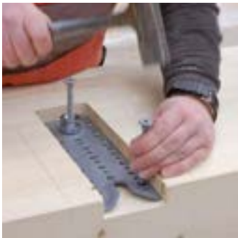
Position the plate and the screws
