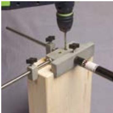
Pre-drill secondary beam
