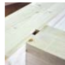
Secured connection using a locking clip
