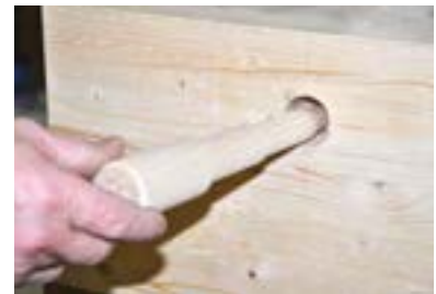
Insert the peg up to the nail head
