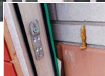
Installation example: WALCO® Z40 mounted on the wall with double-sided element seals.
